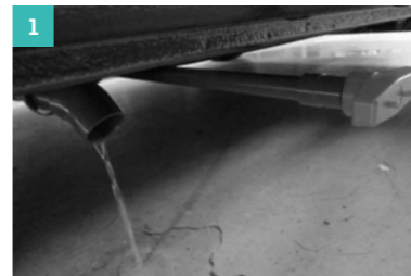
Open the spoil water tank.
